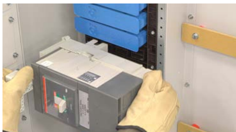
The Breaker Is Inserted Into The SafePanel
